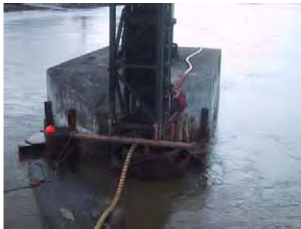
Figure I.11-2c Double-Walled Attenuator – Humboldt Bay Bridges, Eureka, CA
