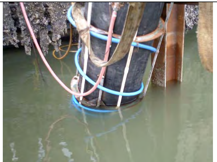
Figure I.4-2b Close-View of Confined Air Bubble Attenuation System next to Vertical H-Type Pile
