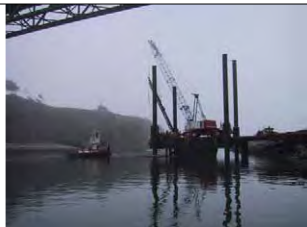
Figure I.4-1b Impact Driving of In-Water H-Type Piles
