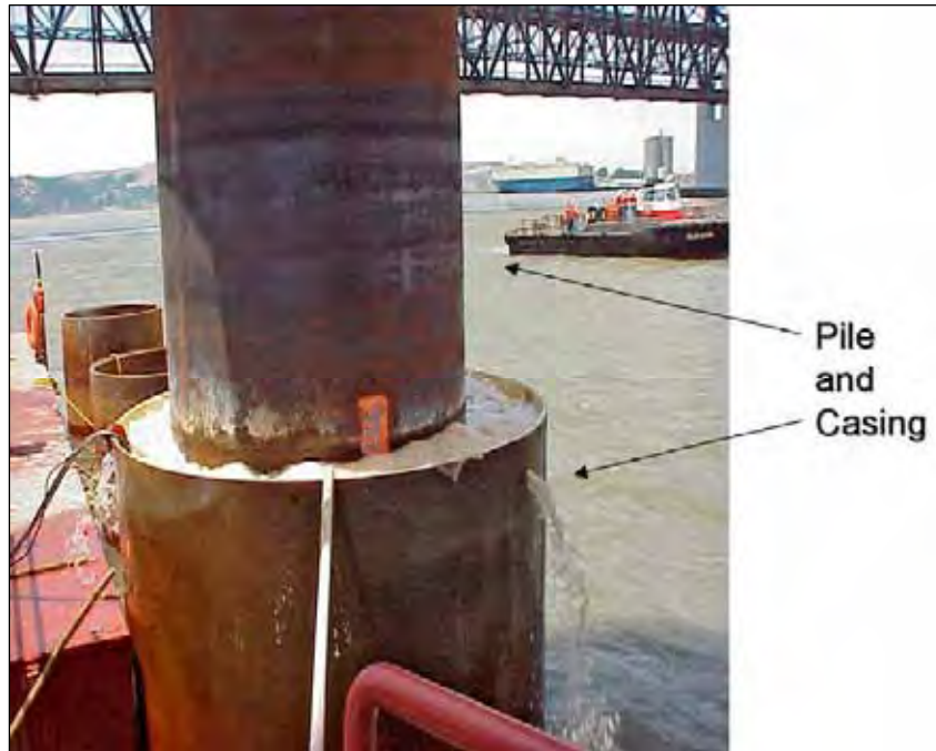
Figure 2-30. Confined Air Bubble Curtain System Used in an Isolation Pile at the Benicia-Martinez Bridge
