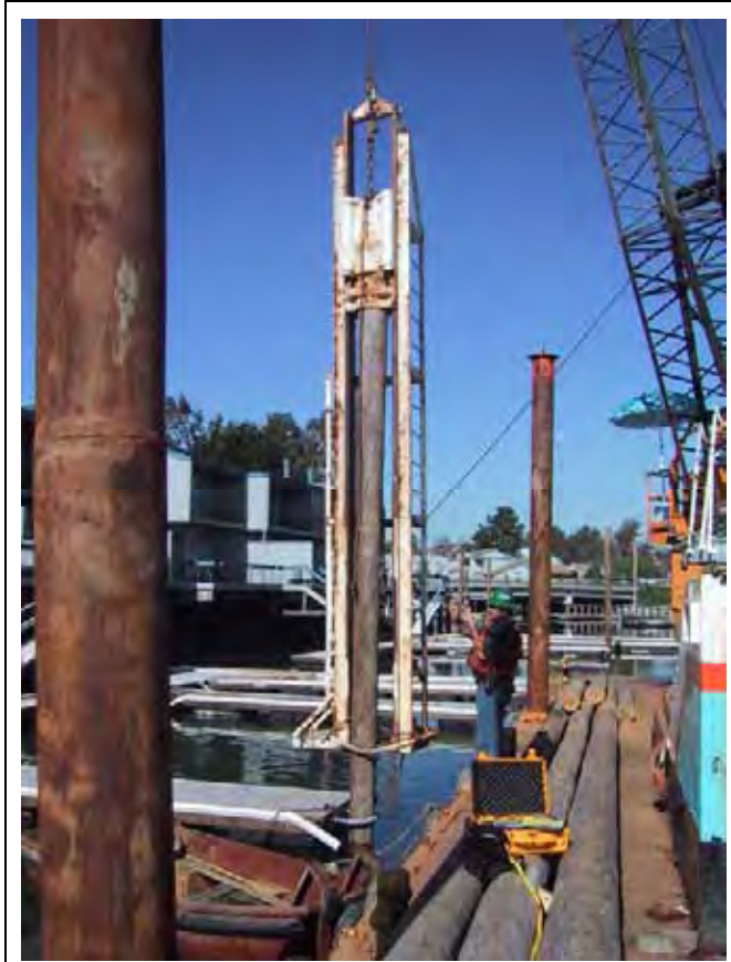
Figure I.7-1 Driving of Timber Piles at Ballena Bay Marina Using a 3,000-Pound Drop Hammer
