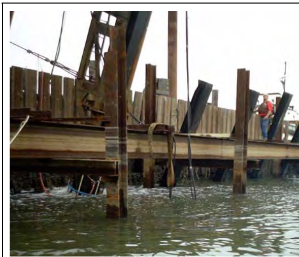
Figure I.4-2a Impact Driving of Battered H-Type Pile with Attenuation System, with Vertical Thin-Walled H-Type Piles in Foreground
