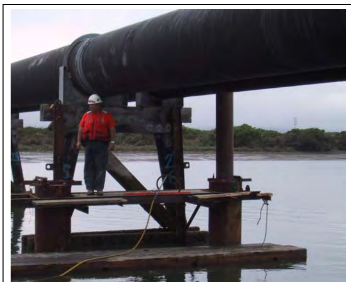
Figure I.3-3 Installation of 13-Inch-Diameter Steel Pipe Piles with Confined Air Bubble Curtain System
