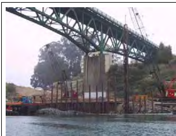
Figure I.4-1a Impact Driving of On-Shore H-Type Piles
