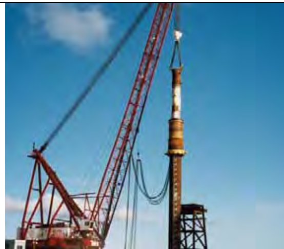
Figure I.9-3b Large Hydraulic Hammer (MHU1700T) Hammer Used for Last Quarter of Pile Driving Where Resistance Was Greatest
