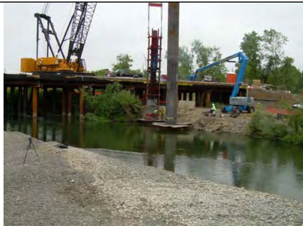
Figure I.3-22b Driving the Top Pile Section of Bent 5 Using a Dewatered Casing to Reduce Sound
