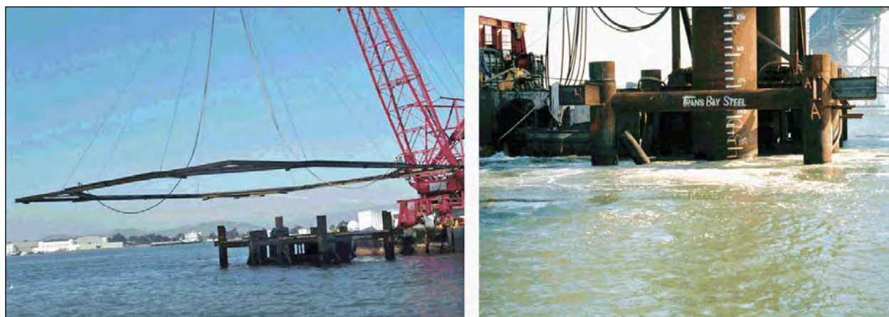
Figure 2-20. Unconfined Air Bubble Curtain Systems
