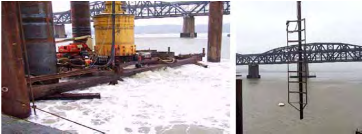
Figure 2-25. Multiple-Stage Unconfined Air Bubble Curtain System
