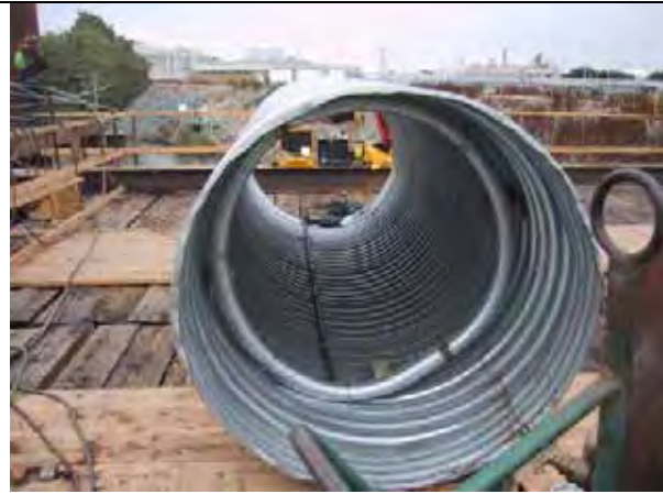
Figure I.3-8 Casing for the Confined Air Bubble Curtain System
