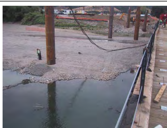
Figure I.3-22a Vibratory Installation of a Bent 4 Pile with Bent 3 and Bent 2 in the Background
