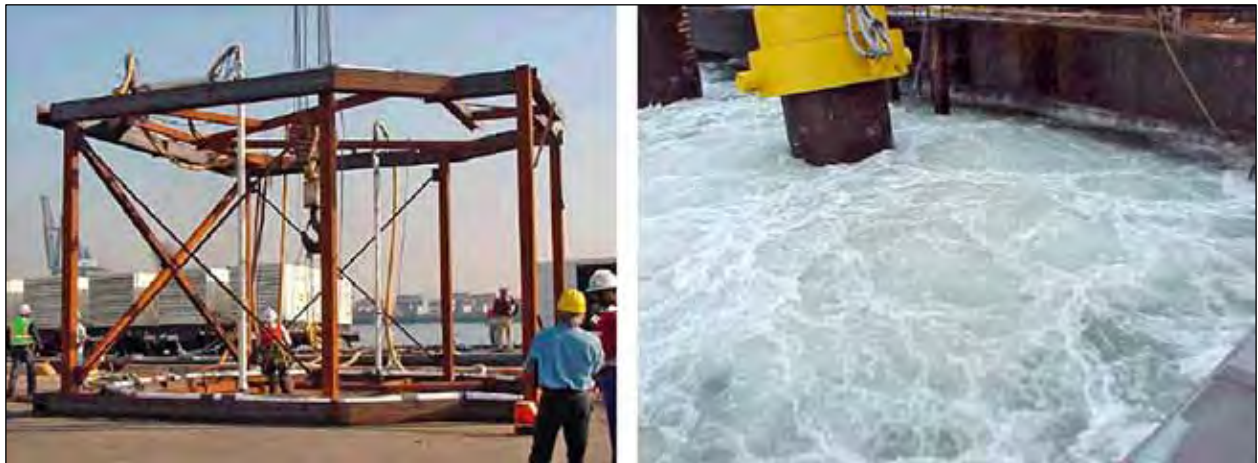
Figure 2-22. Dual-Stage Unconfined Air Bubble Curtain
