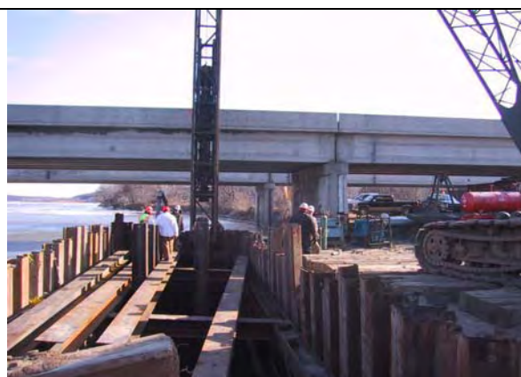
Figure I.4-5b Dewatered Cofferdam Excavated below Water Level
