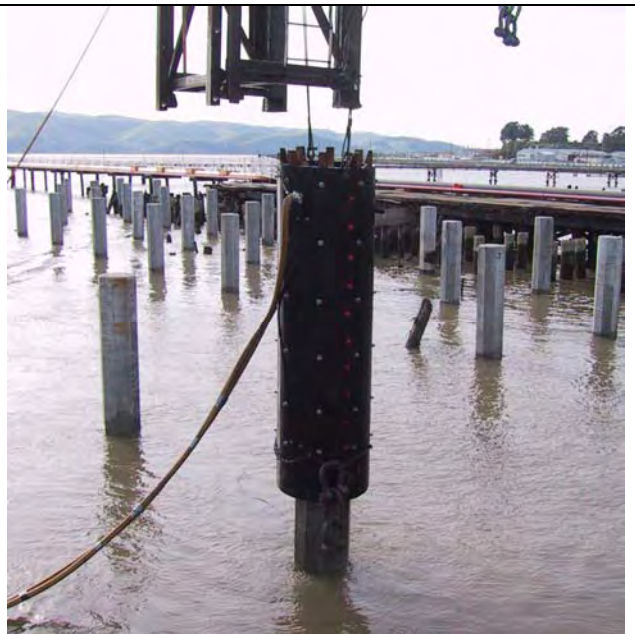
Figure I.5-4b “Bubbleator” Used to Attenuate Underwater Sound
