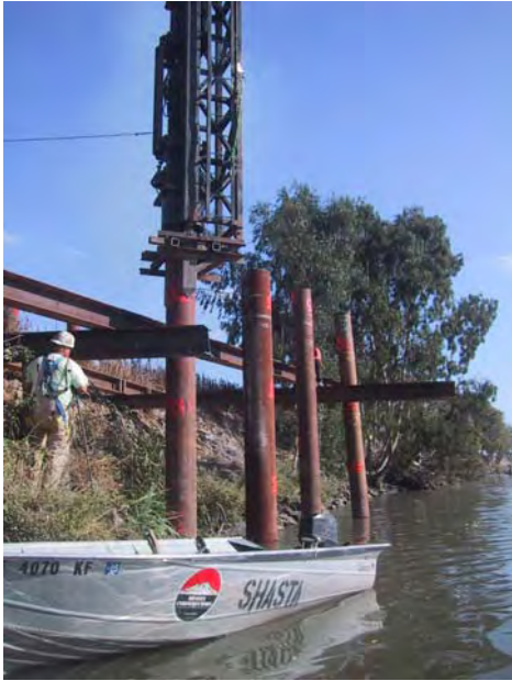
Figure I.3-7a Driving 20-Inch-Diameter Piles near Shore
